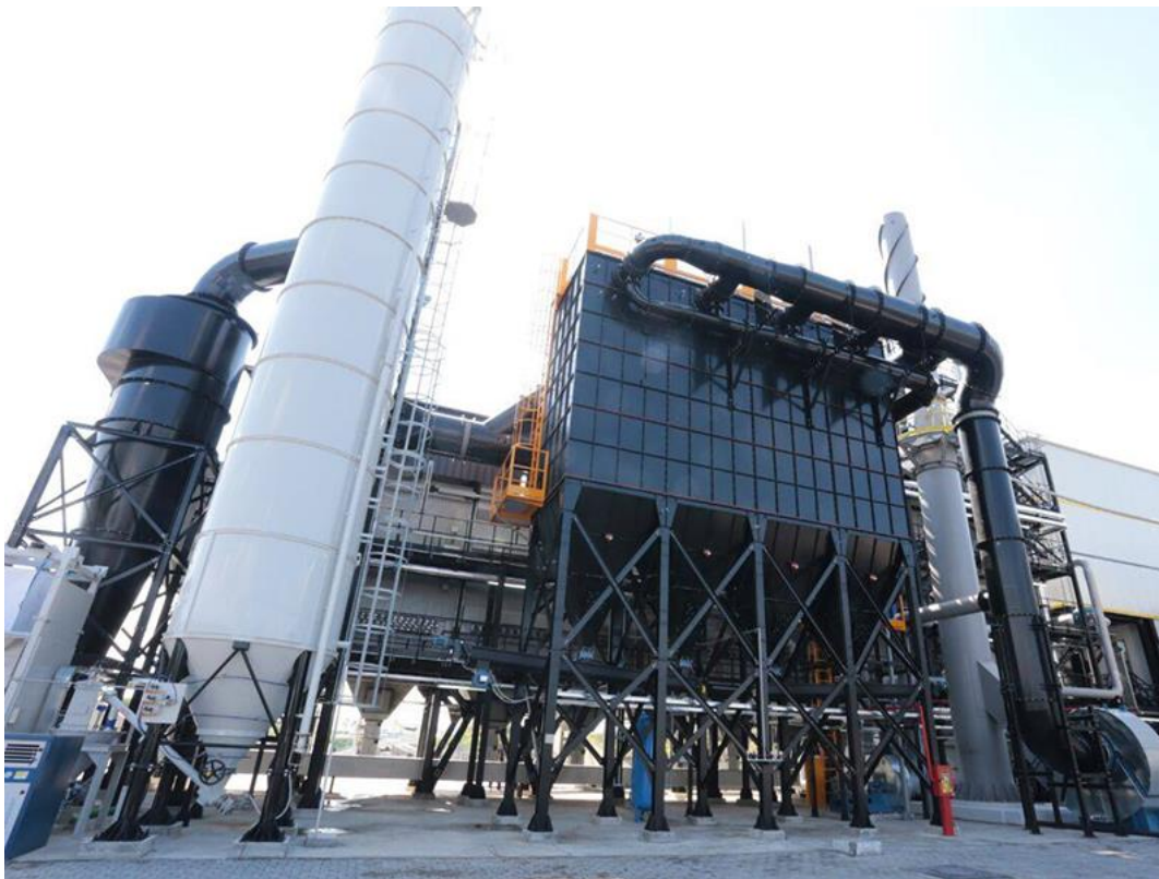
Fig 7 17 View from Energy production plant, Elbasan
