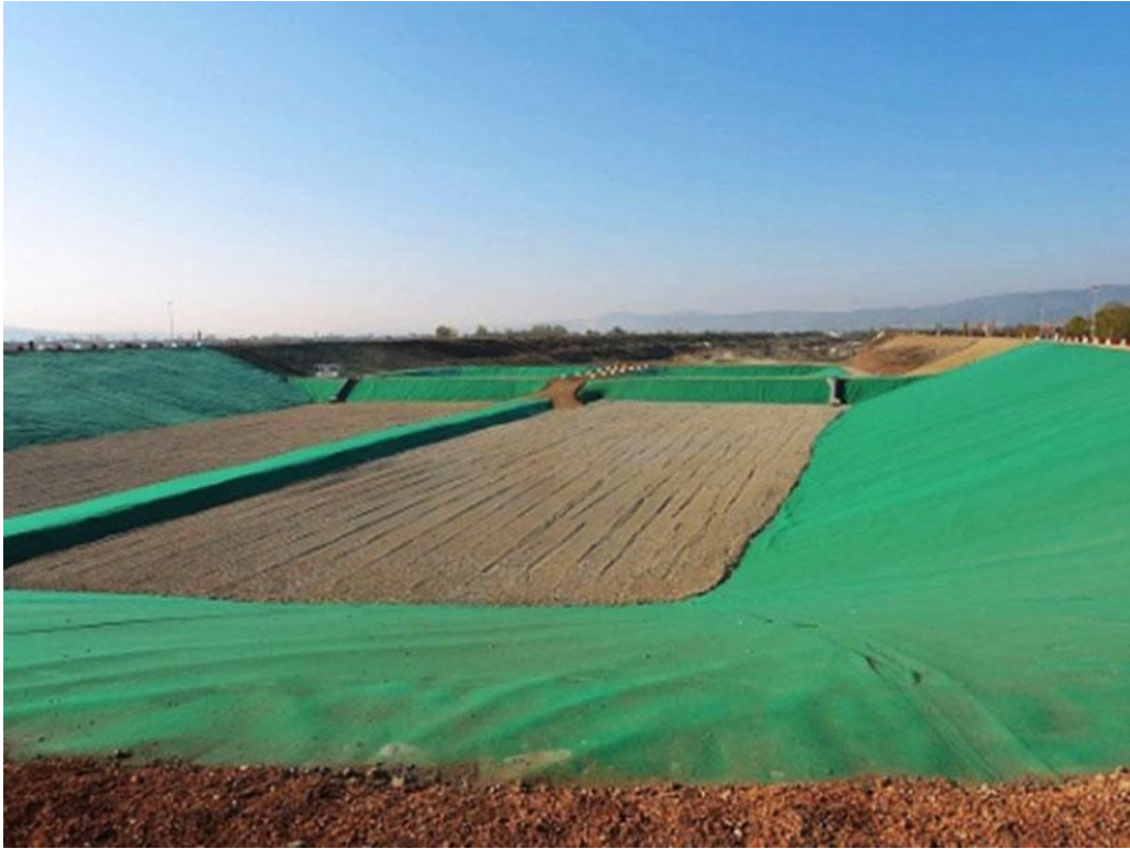
Fig 7 16 View from Elbasan landfill, part of Solid Waste treatment plant
