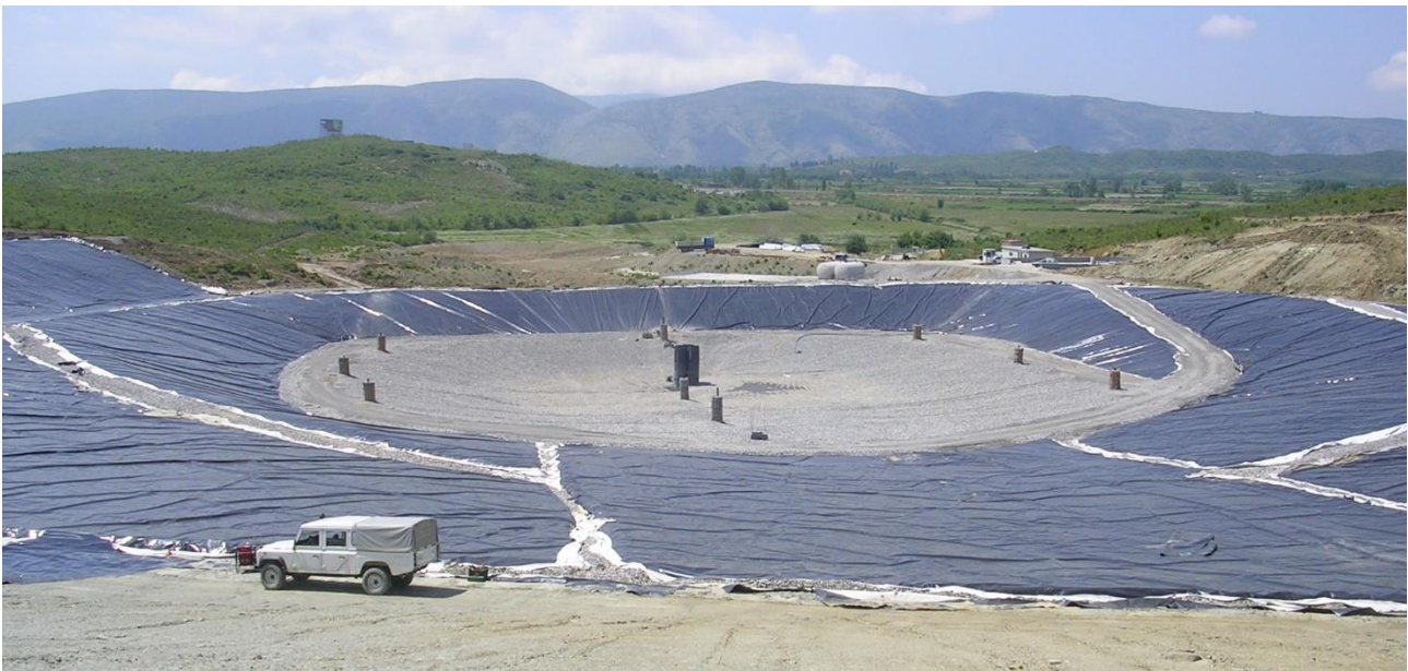
Fig. 7.2 Bushat landfill view
